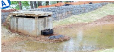
Good construction and operation. Note long basin design, seeded sidewalls, and flow restrictor (half-pipe and rock berm) in front of inlet hale.
