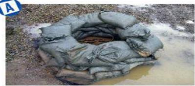
Excellent berm of rock bags protecting drop inlet. Note that bags are only half full of rock, allowing tight fit. Good overlap; no large openings visible.
