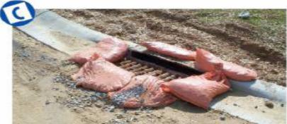
Fair protection of curbside drop inlet. Educate equipment operators on avoiding berms. Use in-drain filters if berms create hazards for roads open to public.
