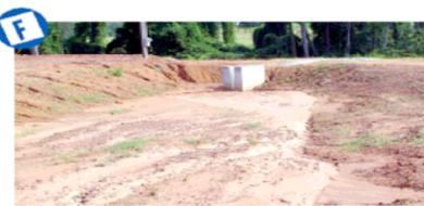
Good length and outlet, but very poor operation and maintenance. Side banks not seeded, no flow restrictor at V-notched inlet. Needs to be deaned out.
