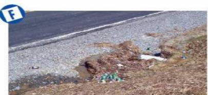
Poor inlet protection-no controls visible. Note straw and debris dogging inlet grating. Rock berms, rock bags, inlet filters, or other products could be used here.
